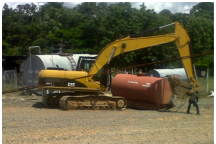
Fuel tanks and excavator
